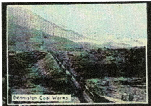
"Denniston Coal Works"
