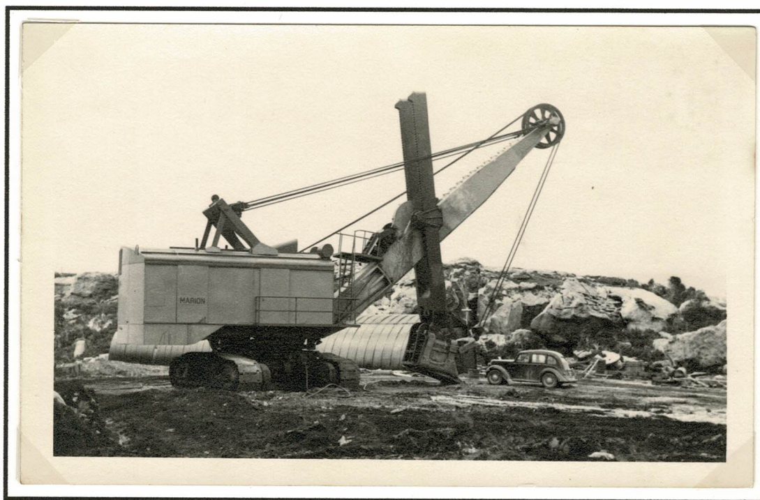
Real photo postcard by R S Richards of Christchurch showing the Marion Shovel dwarfing a car c 1950 . This was the first heavy machinery at Stockton. This steam powered shovel was used to strip overburden. It saw little use and was sold to be used on the Buller River breakwaters
