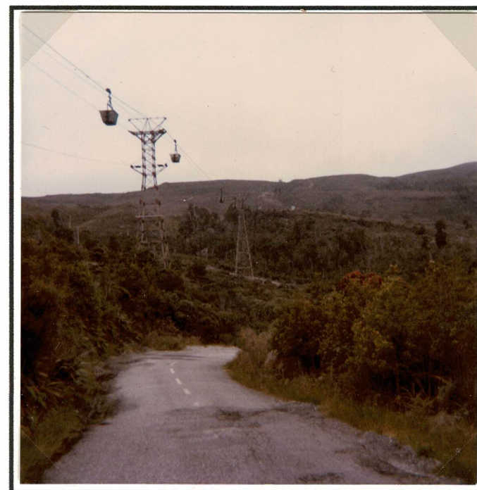
Exhibitor photograph [1984] showing Aerial ropeway - upgraded by State Coal to carry up to 4000 tons a day
