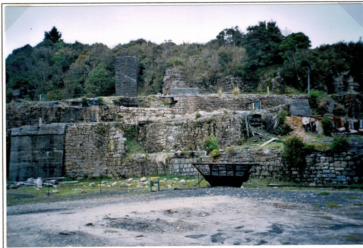
Above: The Brakehead c 1950 with the extended bins and conveyor belt and loading chute in centre with 2 loaded wagons at left ready to descend the Incline and an empty on the right Photo reproduction Coal Museum Westport
