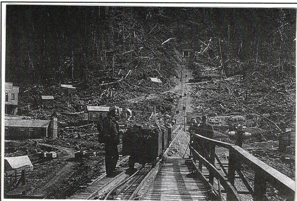
Roa Mine - incline ropeway haulage to Mine [from "Grey District Coal Mining in Photographs" History House 2015]
